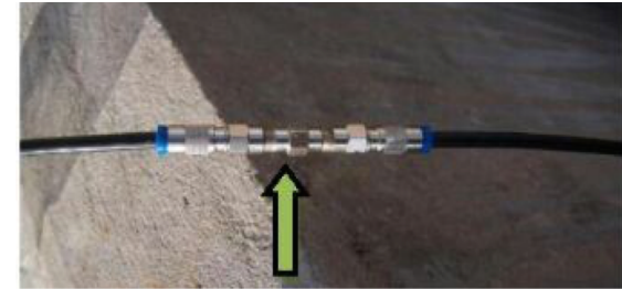
Bare Connector Joint
